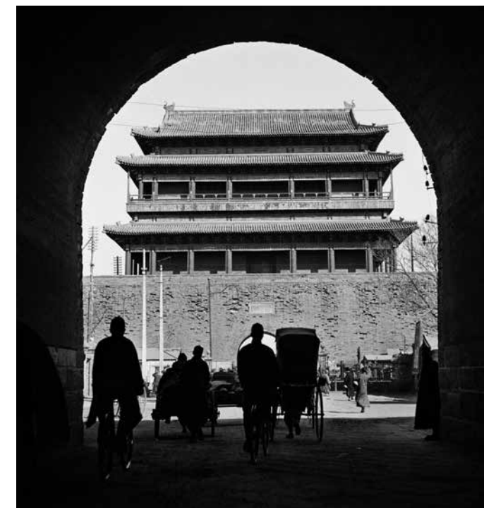
Chongwenmen poort, Beijing, China, 1931-1934 © Ellen Thorbecke
